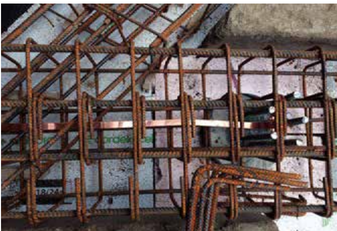
The steel reinforcement itself is bonded into the building's earthing/lightning protection; the bright copper strip can be seen fixed to the steel
