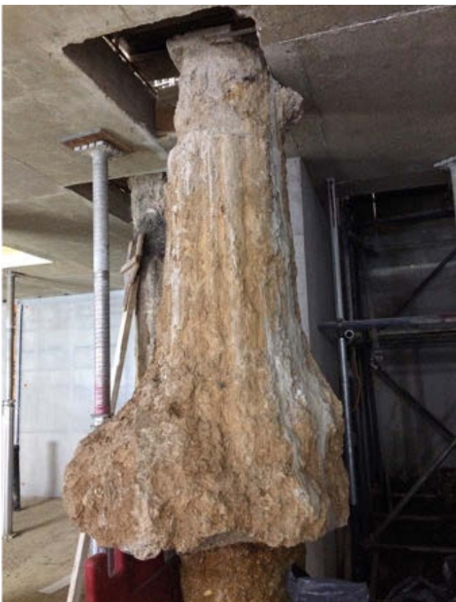
A remaining sacrificial pile within the new basement to be removed, bearing a remarkable resemblance to a calcified elephant's foot!
