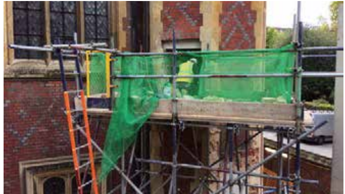
The new entrance being cut into the old North West tower. Note the concrete beams over the new opening. Due to the thickness of the brickwork in this location, several beams were needed in a carefully sequenced operation
