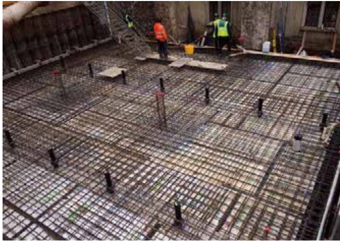
After the bearing piles and piled walls were completed, the formwork and steel reinforcement was set out for the floor slabs, ready for concrete pouring. Above and below are photographs before and after the concrete pour
