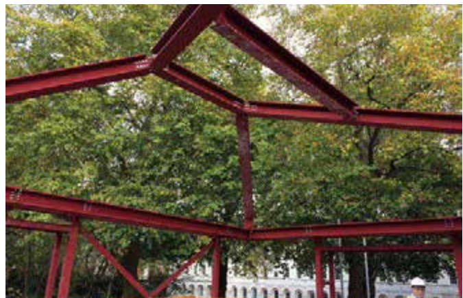
The reinforced concrete frame has now been completed and the blockwork walls are currently being constructed. The roof steels are in place awaiting the joists, ply diaphragm and lead covering
