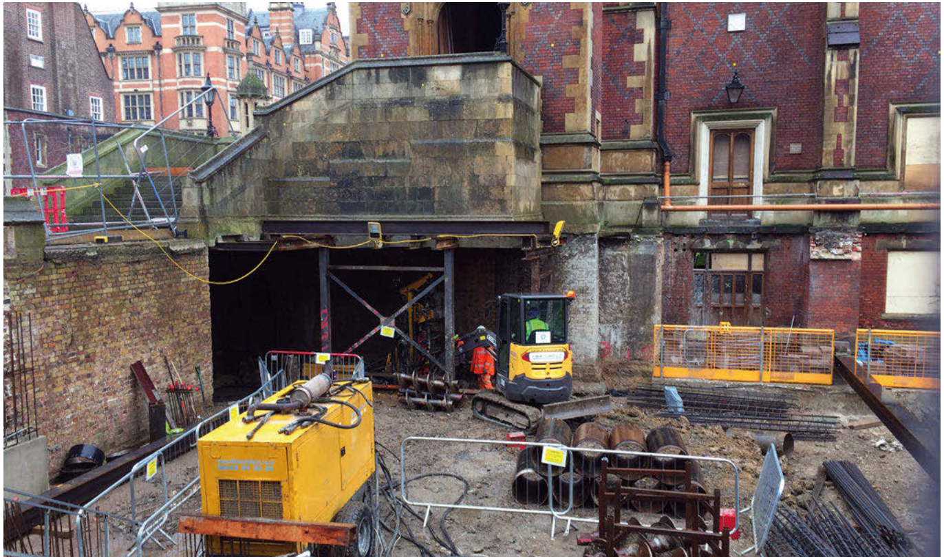
The 'floating' staircase supported by temporary steelwork. To the right of the man in the orange hi-vis jacket is the mini-piling machine, and to his left are auger bits ready for successive installation. There are more auger bits in the foreground
