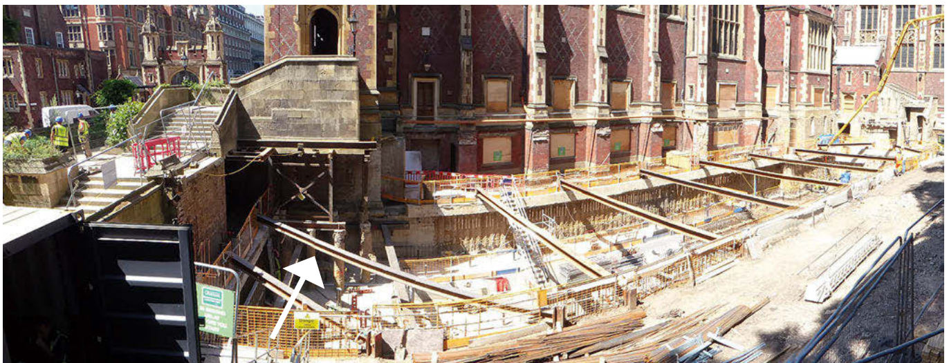
The sacrificial piles can be seen under the temporary steelwork
