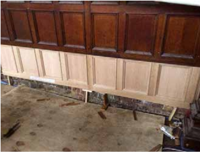
The old perimeter heaters in the Great Hall have been removed, and new hardwood panelling to match has been fixed below the existing panelling. Once the RH and temperature have stabilised, these panels will be stained and French polished to match as closely as possible the original panelling
