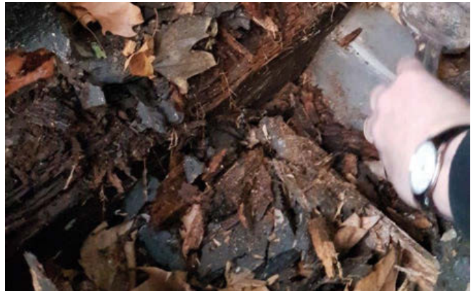
A rotten timber joist in the Old Hall roof
