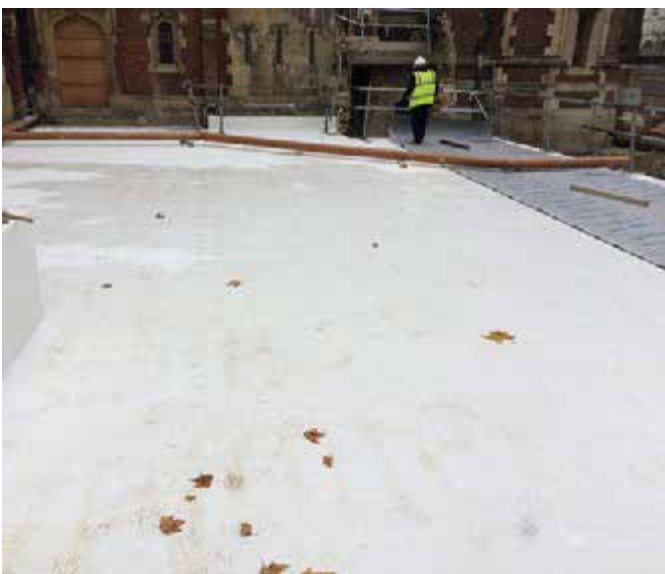
The first of the waterproofing layers being applied to the East Terrace
