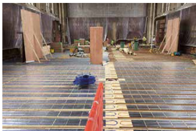
The Great Hall part way through the under-floor heating installation and floor renewal
