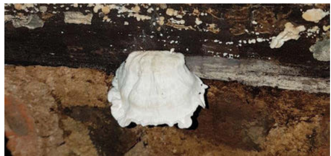
Coniophora (C. puteanan) . Commonly referred to as the wet rot fungus in the Old Hall bay window roof wall plate
