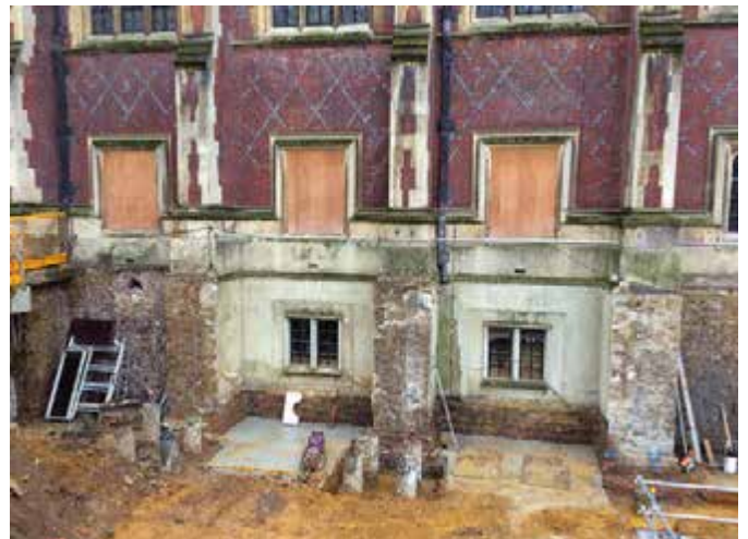
A rarely seen view of the existing Library basement windows, after the retaining walls, which formed the light wells for the windows, were demolished. These will form access openings through to the new Library basement
