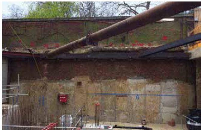
The excavation for the Library basement had been preceded by underpinning the boundary wall. In the view above, taken after both the underpinning and excavation was completed, an earlier wall can be seen between the new concrete underpinned sections and the early Victorian perimeter wall. The project archaeologist believes this was built around 1500-1550
