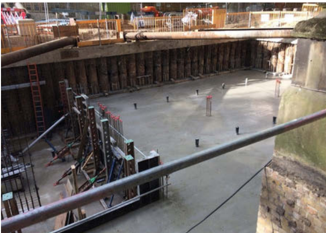
After the bearing piles and piled walls were completed, the formwork and steel reinforcement was set out for the floor slabs, ready for concrete pouring. Above and below are photographs before and after the concrete pour
