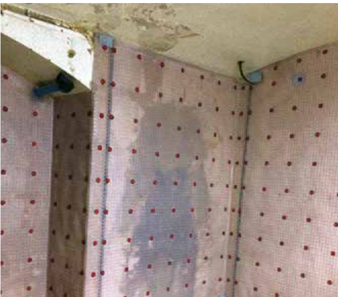
The drained waterproofing system can be seen here fixed to the wall. Behind is the ghostly image of an old solid fuel cooker from generations ago
