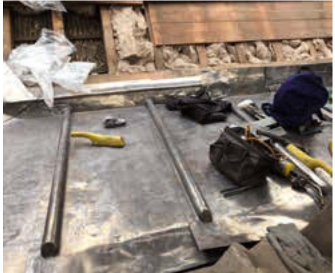
Lead roofs were also renewed where needed.
