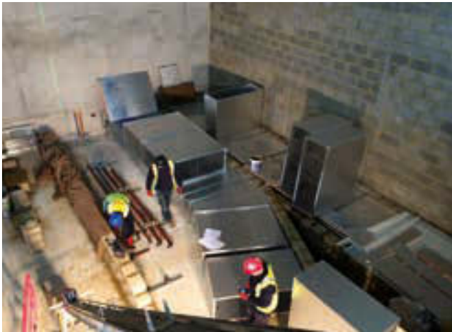
Underfloor ducting and sleeper walls being formed in the lecture theatre.
