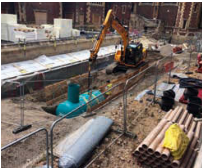
The green rainwater harvesting tank lowered into position.
