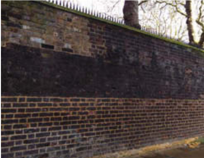
The boundary wall prior to repairs. Spalling brickwork, decaying rendered plinth, dirty brickwork and failed pointing can be seen.
