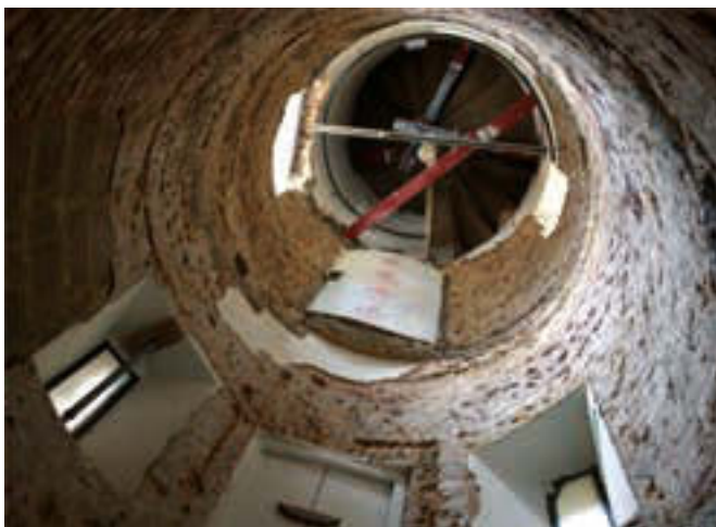
The North West Tower with the staircase removed. The temporary steelwork supporting the remainder of the spiral staircase over can clearly be seen.
