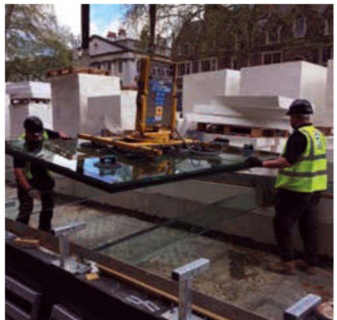
The glazing units for the central rooflight being manoeuvred into position.
