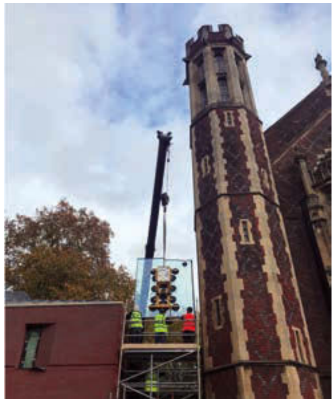
Right: The link bridge glazing being craned into place.
