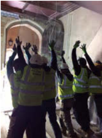
The glass door being raised into position.
