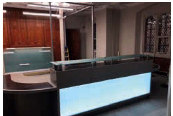
The new reception area, with the new partition frames awaiting glass fitting.
