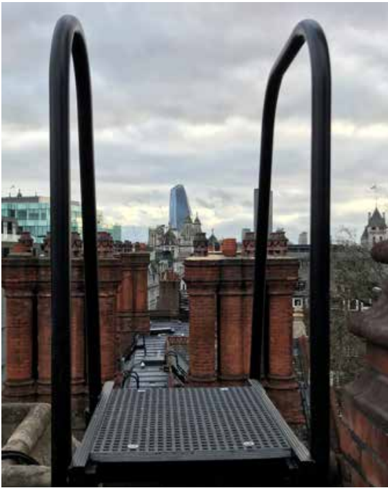
The replacement roof access equipment was much more sturdy
