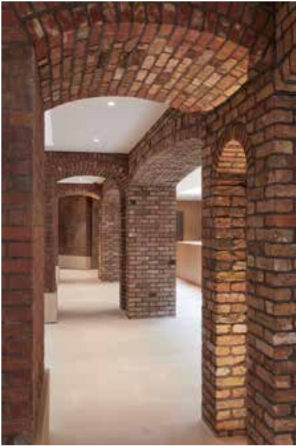
A view of the below ground break-out spaces, previously external space which provided the lightwell for the kitchen windows and the retaining wall for the East Terrace.
