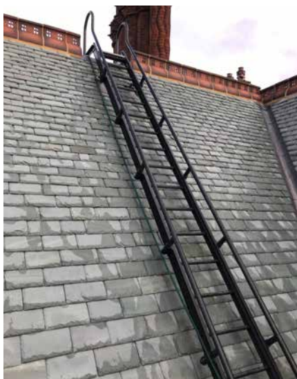
The new roof, with new access ladders
