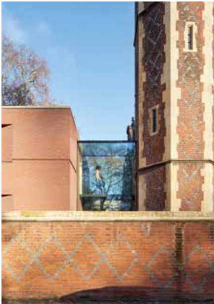
A view of the bridge linking the library extension and main building. This uses structural glass of low iron content to minimise reflections and maximise the view through the glass from the outside.
