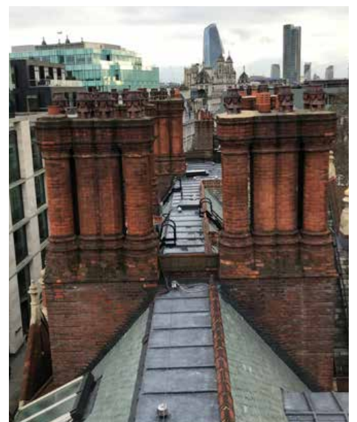
New lead roof bays above the slate roof
