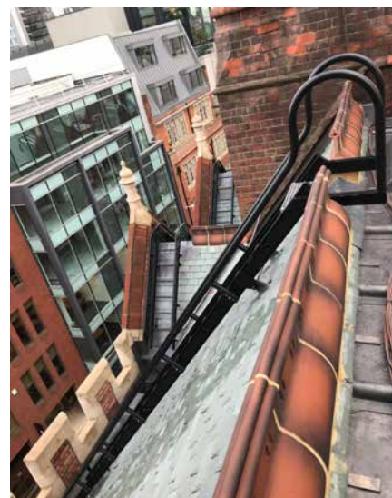
Another view of the roof showing the new clay ridge tiles and the troublesome gables
