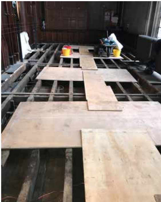
The Minstrels Gallery in the Great Hall was suffering from excessive deflection. Removal of floor boards and ply facilitated inspection, and showed a number of historic defects, which were resolved by the installation of additional joists and improved fixings.
