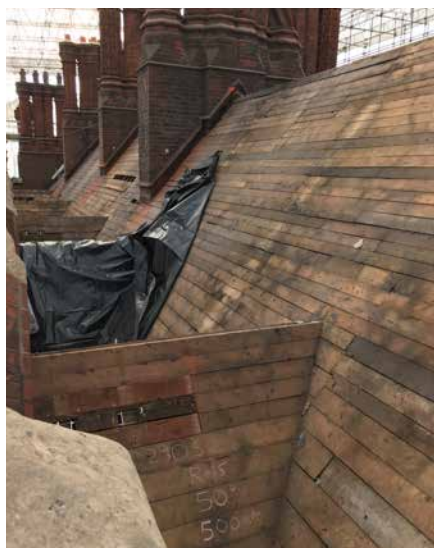
The close-boarded roof after the slates have been removed
