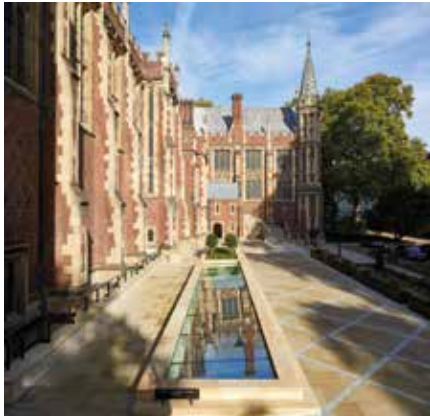
The roof lights have been set in a stone surround, doubling as external seating, which compliments the new granite stone flooring to the East Terrace, set diamond pattern in the York stone paving. This reflects the diagonal brick diapering of the Great Hall walls in a style also used on the Thames terraces in the Palace of Westminster.
