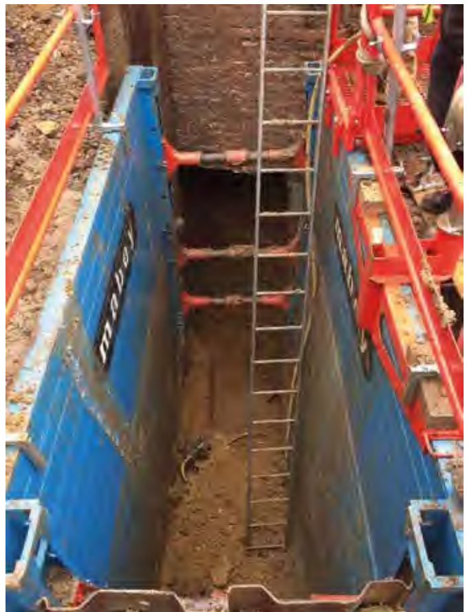
The void opened up under the boundary wall, which was subsequently filled with brick and concrete to underpin the wall.
