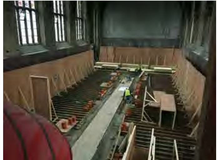
View of the Great Hall from the Minstrels Gallery showing panelling protection
