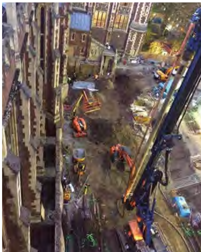
This view shows the 20m piling rig in operation together with earth moving plant and a cherry picker
