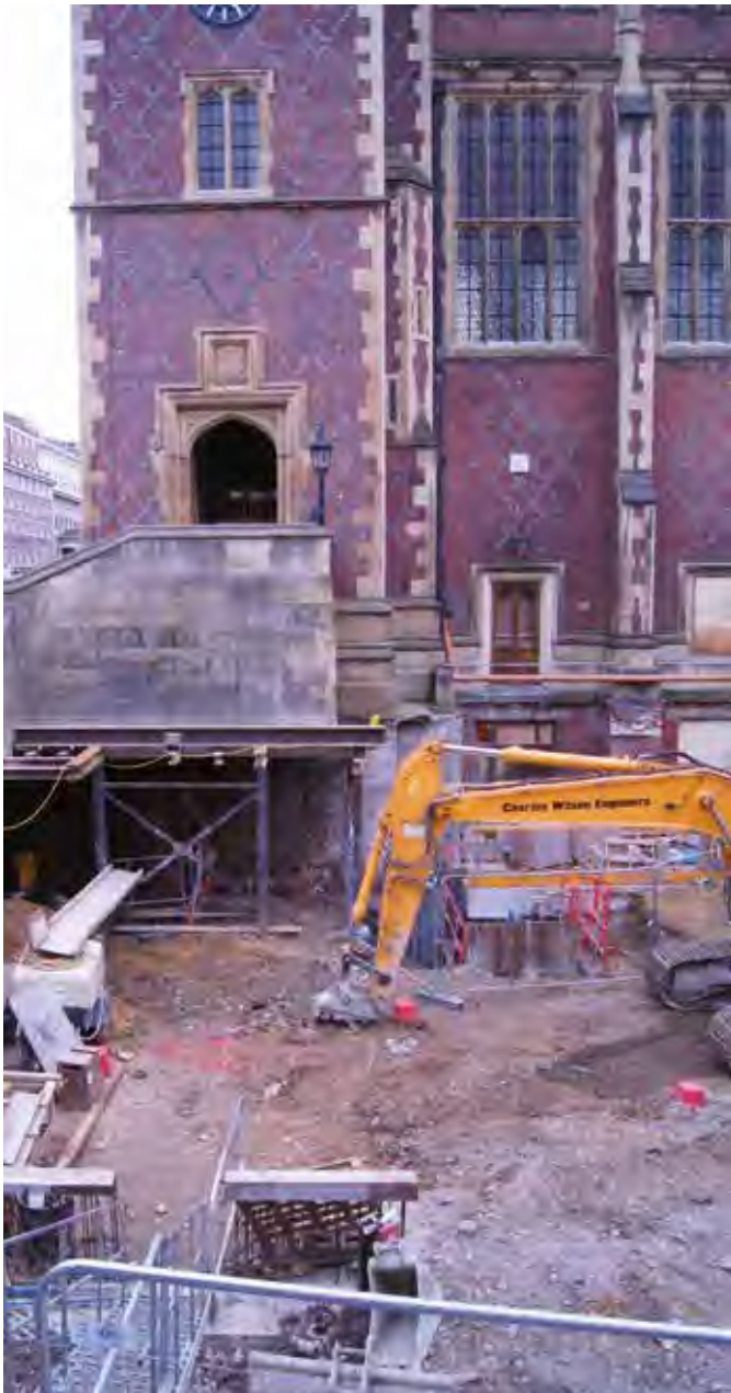
Steel grillage supporting the “floating” ceremonial staircase, allowing demolition of the supporting brick wall, needed to make space for the Education basement extension
