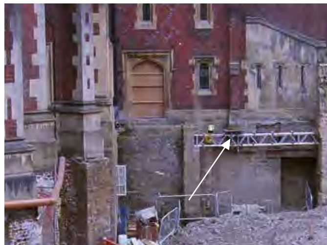
The reduced level dig to the first basement level. The brick buttress to the junction of the library vestibule/stairs was found to be entirely unsupported and was built directly off the paving
