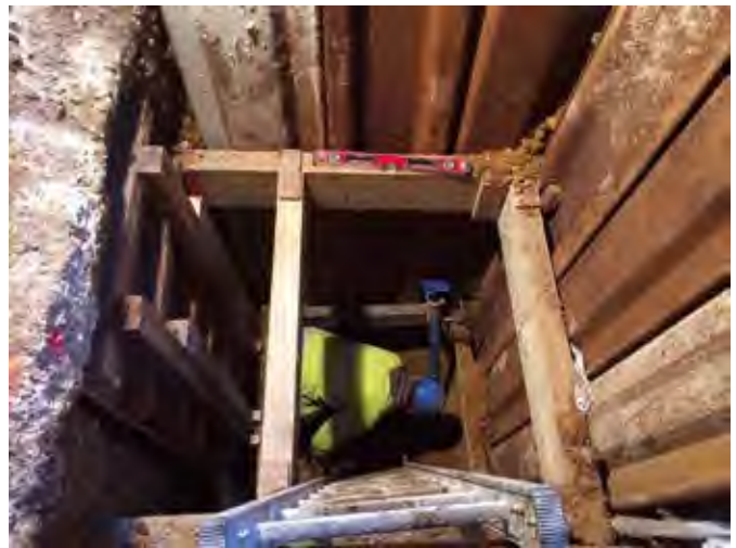
Underpinning the Clocktower
