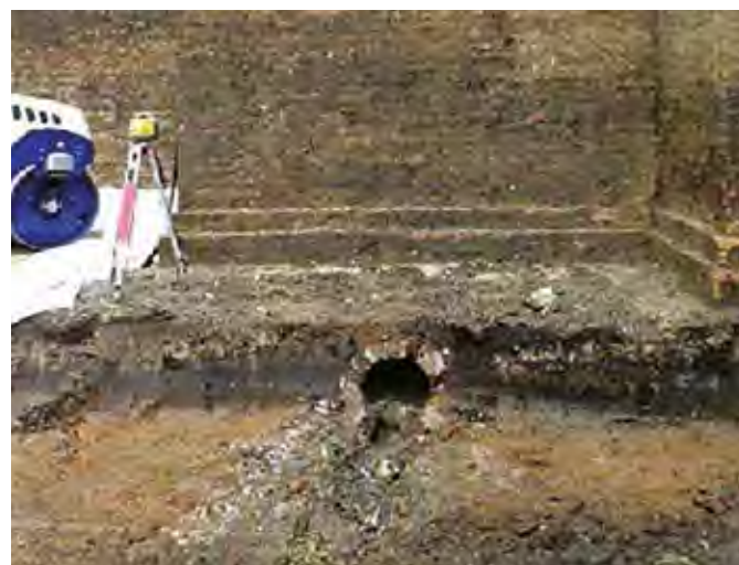
The shortly to be re-opened South ceremonial staircase, supporting brickwork and drain underneath
